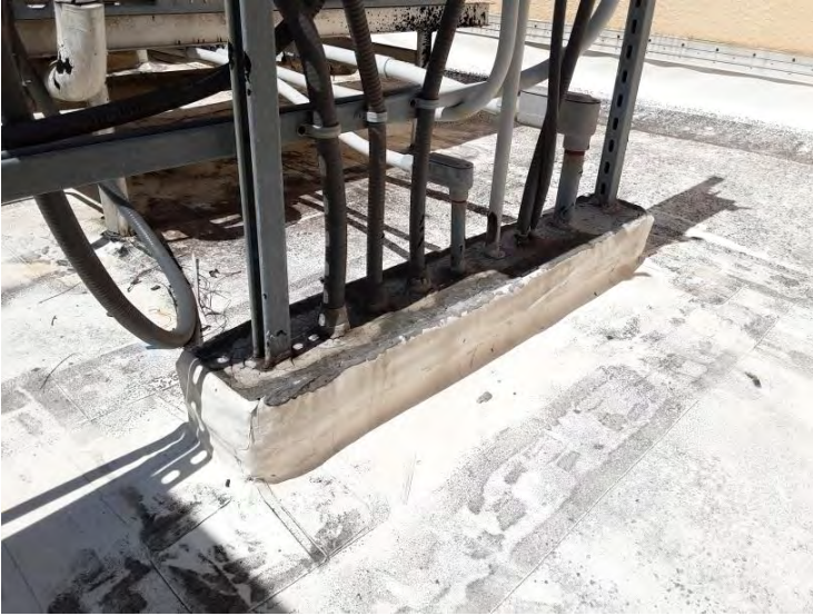
North TPO Roof - Pitch Pans
