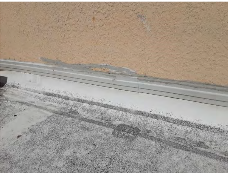
South TPO Roof - Counter Flashings
