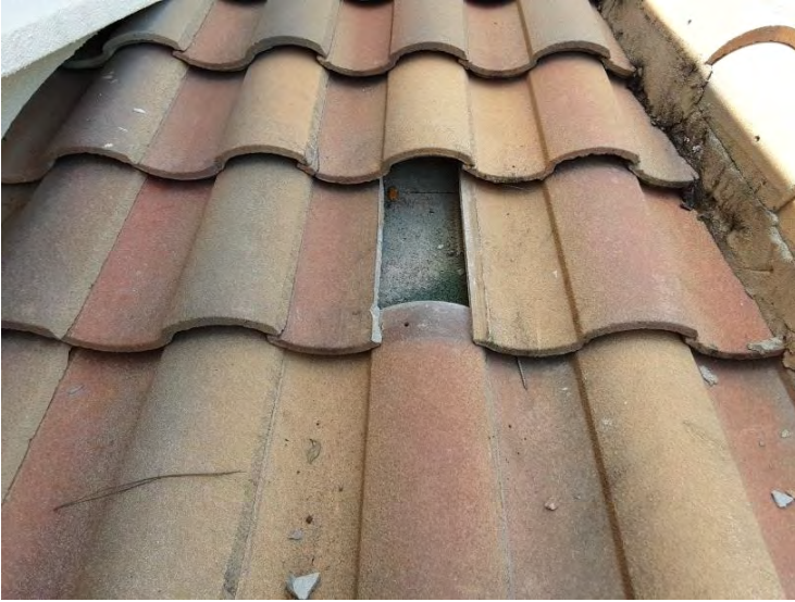
Center Tile Roof - Field Tiles - Damaged Tiles
