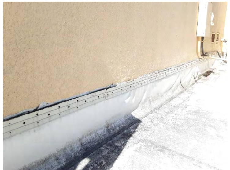
North TPO Roof - Counter Flashings
