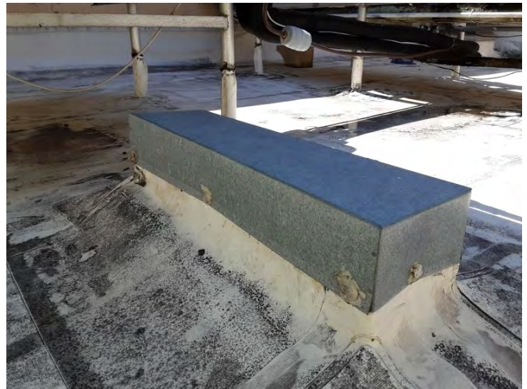
North TPO Roof - Curb
