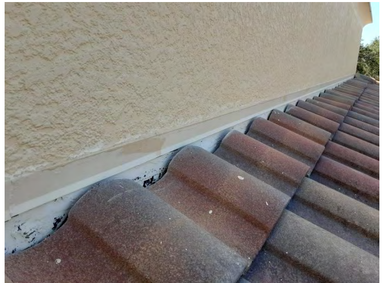
South Tile Roof - Counter Flashings
