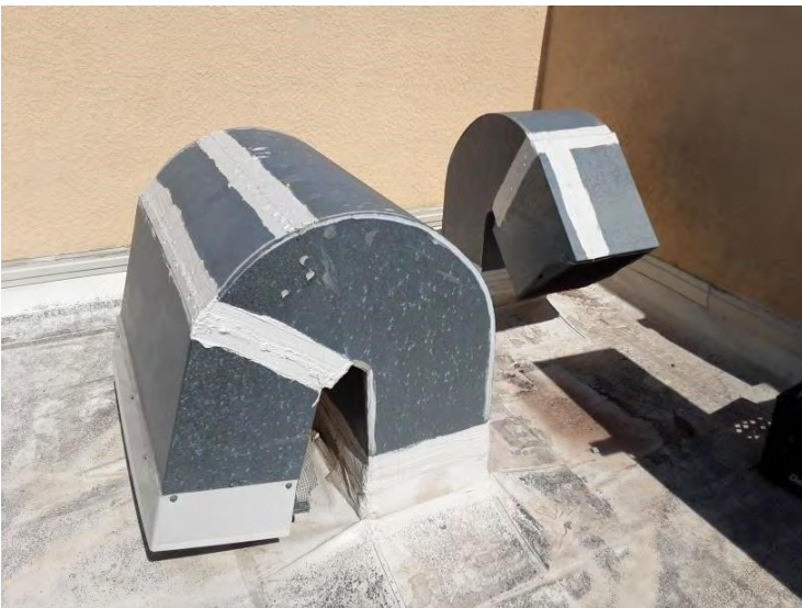
South TPO Roof - Roof Vents Roof vents appear to be in fair condition.
