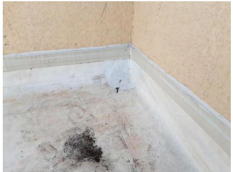
South TPO Roof - Counter Flashings
