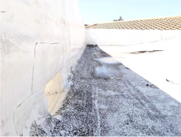
Center TPO Roof - Base Flashings
