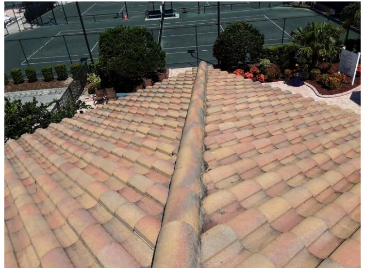
North Tile Roof - Hip Tiles Hip tiles appear to be in fair condition.
