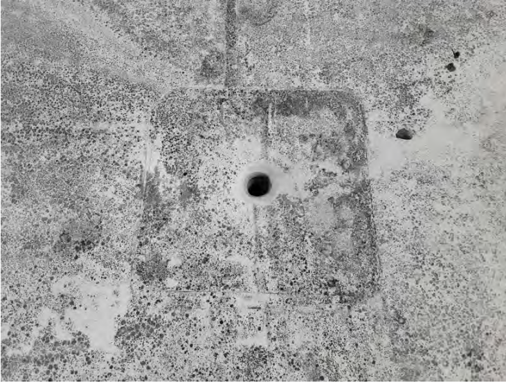
Center TPO Roof - Roof Drains Roof drains appear to be in fair condition.
