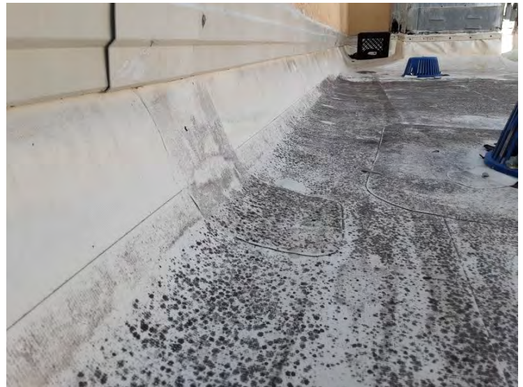
South TPO Roof - Base Flashings
