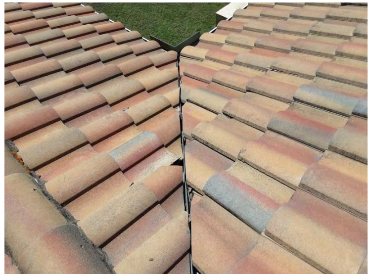
North Tile Roof - Ridge Tiles Ridge tiles appear to be in fair condition.
