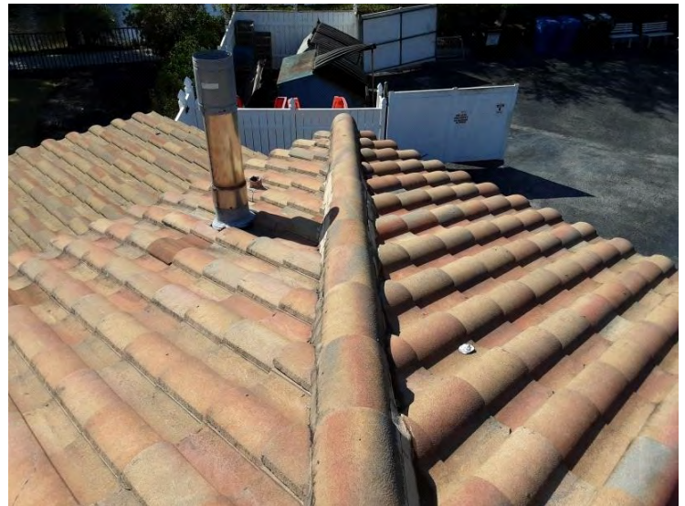
South Tile Roof - Hip Tiles Hip tiles appear to be in fair condition.
