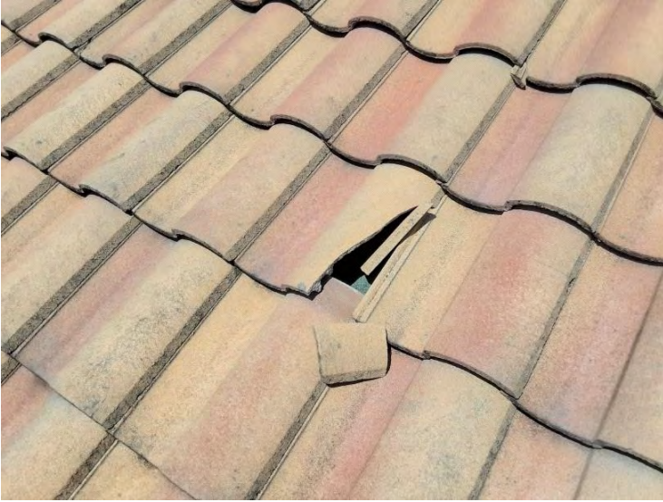
North Tile Roof - Field Tiles - Damaged Tiles
