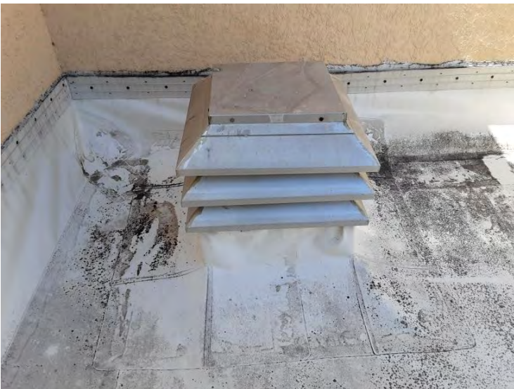
North TPO Roof - Roof Vents Roof vents appear to be in fair condition.
