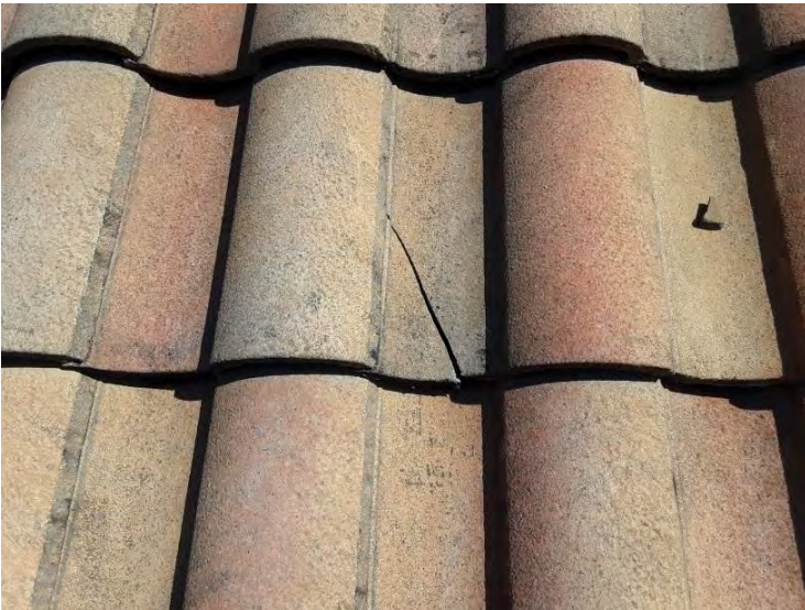
South Tile Roof - Field Tiles - Damaged Roof Tile
