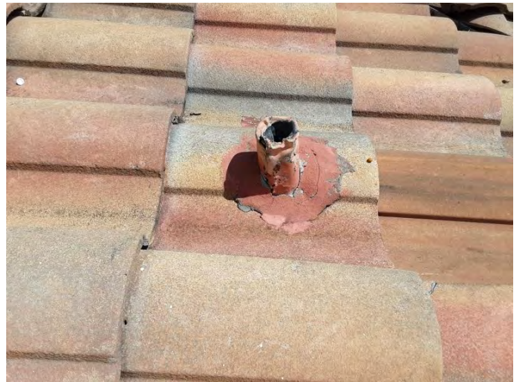
South Tile Roof - Lead Boots Lead boots appear to be in fair condition.
