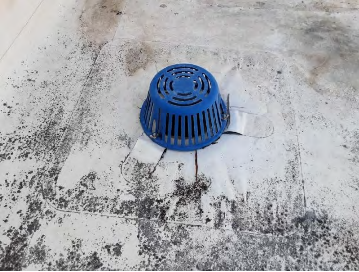
South TPO Roof - Roof Drains Roof drains appear to be in fair condition.
