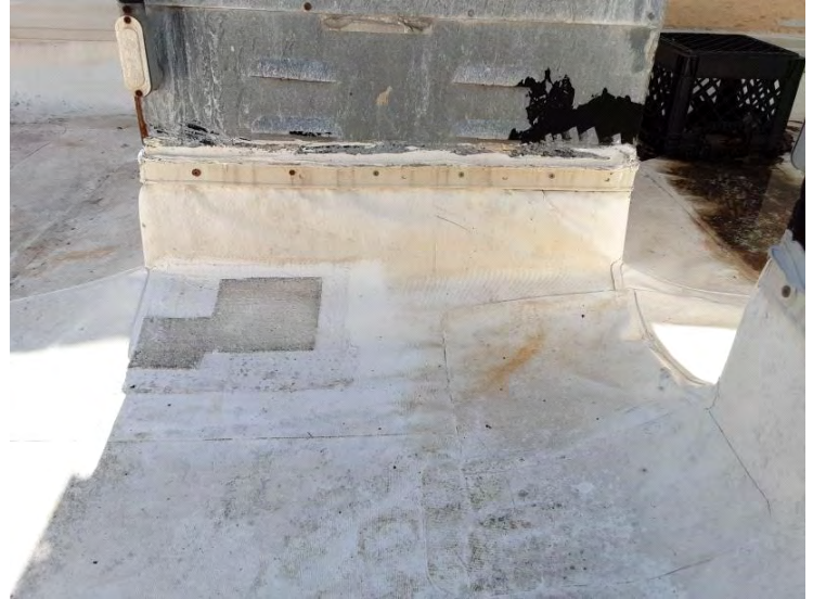
South TPO Roof - Roof Vent Base Flashings Roof vent base flashings appear to be in fair condition.
