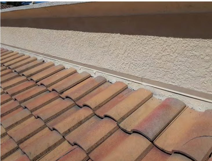
North Tile Roof - Counter Flashings
