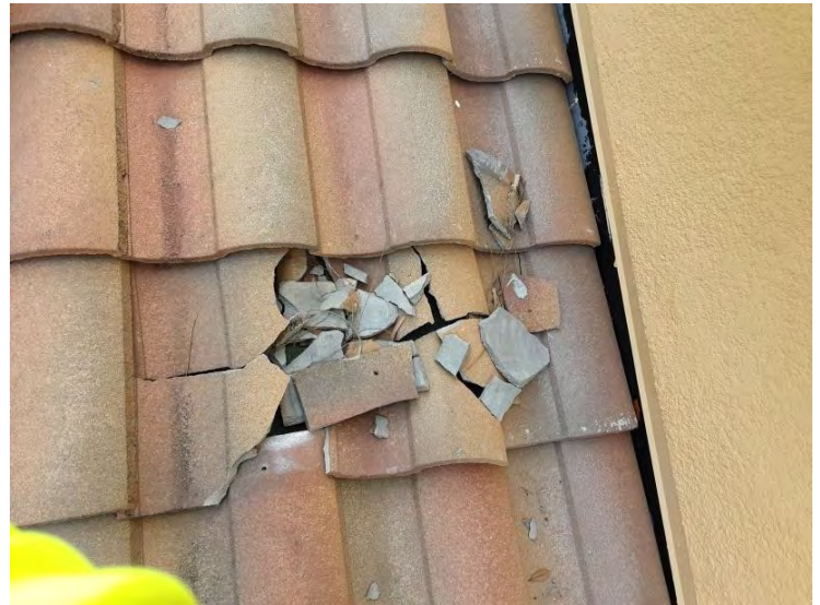
Center Tile Roof - Field Tiles - Damaged Tiles
