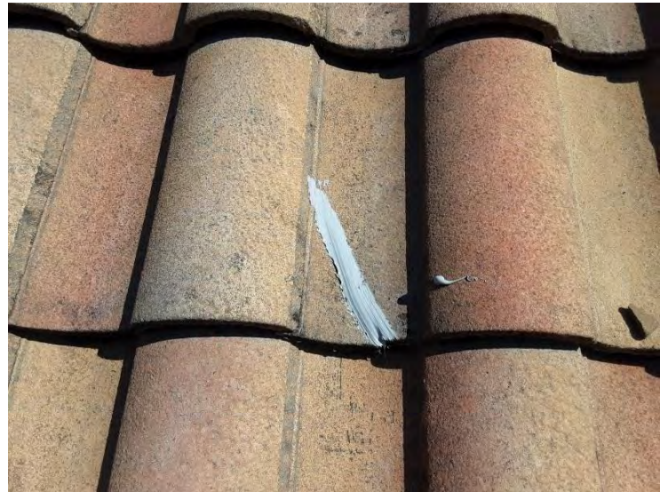
South Tile Roof - Field Tiles - Completed Repair
