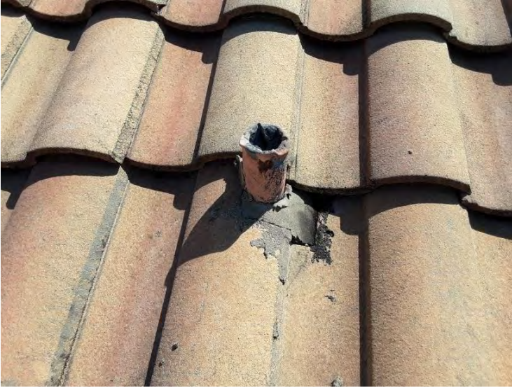
South Tile Roof - Lead Boots Lead boots appear to be in fair condition.
