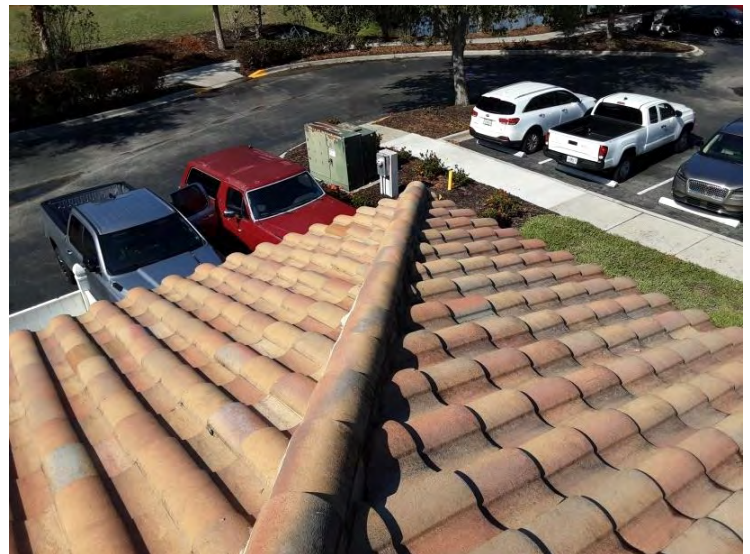
South Tile Roof - Hip Tiles Hip tiles appear to be in fair condition.
