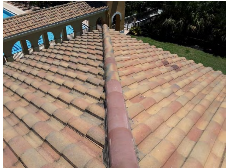
Center Tile Roof - Hip Tiles Hip tiles appear to be in fair condition.
