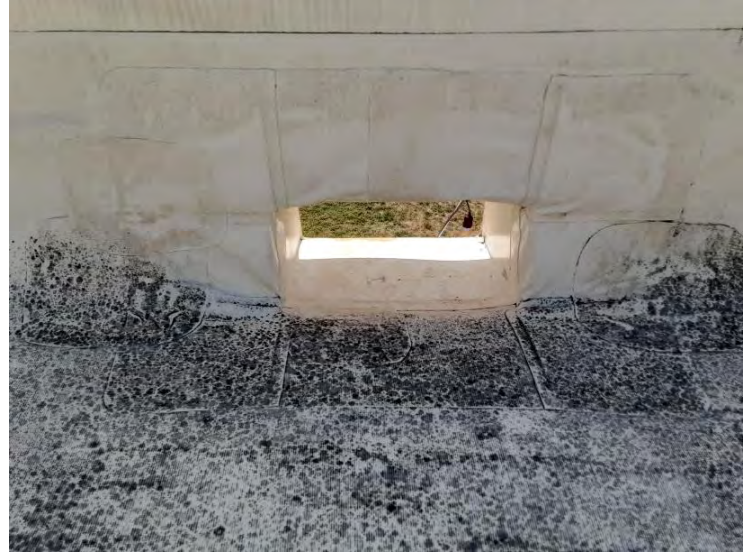
Center TPO Roof - Scupper Scupper appears to be in fair condition.
