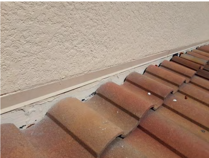
South Tile Roof - Counter Flashings
