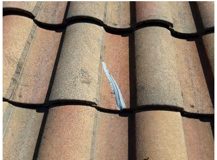
South Tile Roof - Field Tiles - Completed Repair
