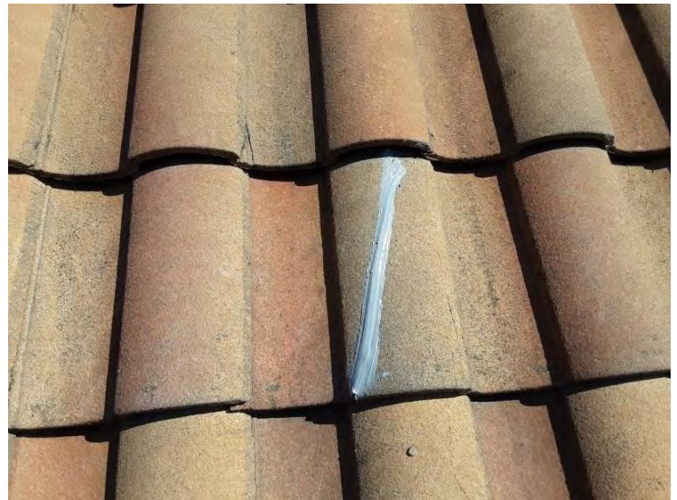
South Tile Roof - Field Tiles - Completed Repair Repaired damaged roof tiles with RT600 sealant.
