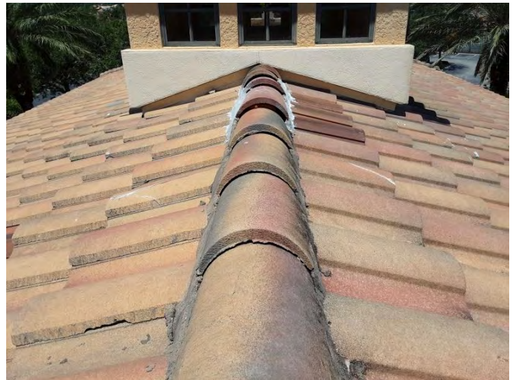
Center Tile Roof - Ridge Tiles Ridge tiles appear to be in fair condition.
