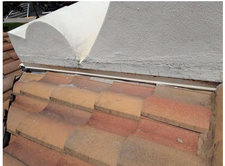
Center Tile Roof - Counter Flashings
