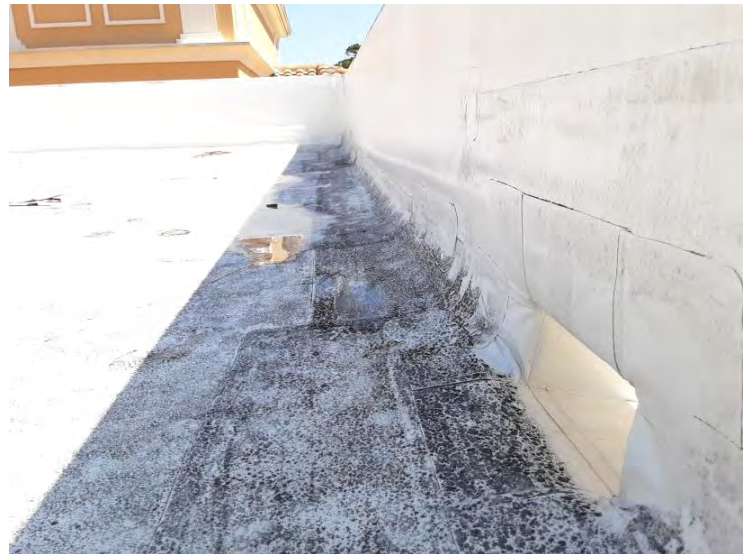
Center TPO Roof - Base Flashings
