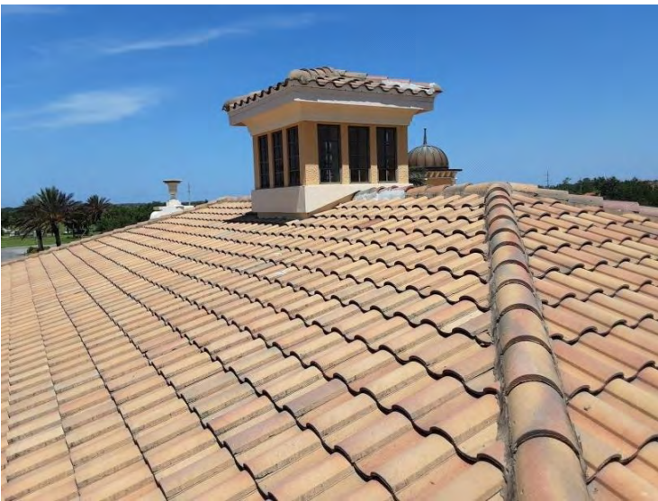
Center Tile Roof - Appearance Overview The appearance of the roof is in fair condition.
