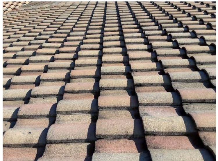
South Tile Roof - Appearance Overview The appearance of the roof is in fair condition.
