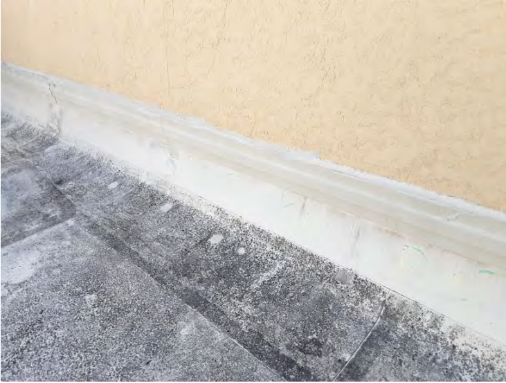
South TPO Roof - Counter Flashings
