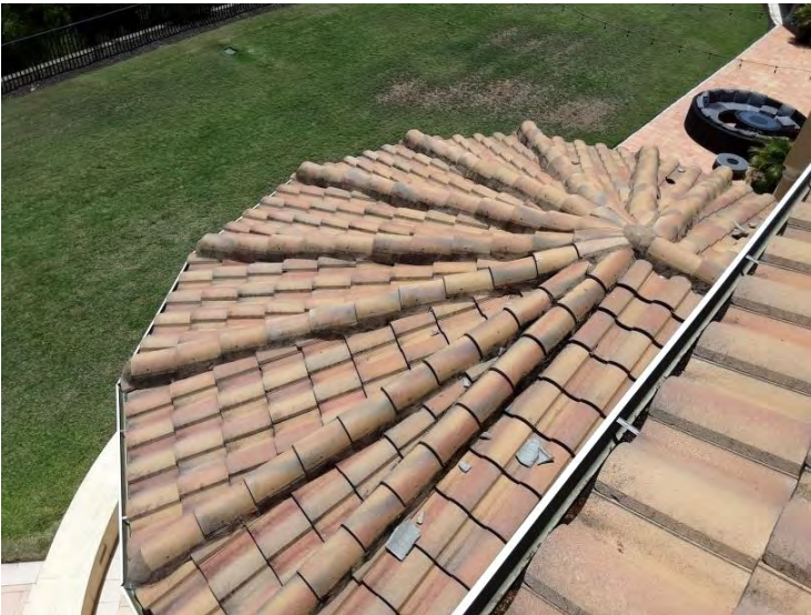
Center Tile Roof - Lower Tile Roof - Appearance Overview The appearance of the roof is in fair condition. Crowther Roofing identified damaged roof tiles.
