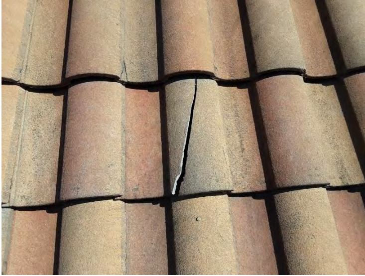
South Tile Roof - Field Tiles - Damaged Roof Tile Identified damaged roof tile that can allow premature underlayment deterioration from excessive UV exposure.
