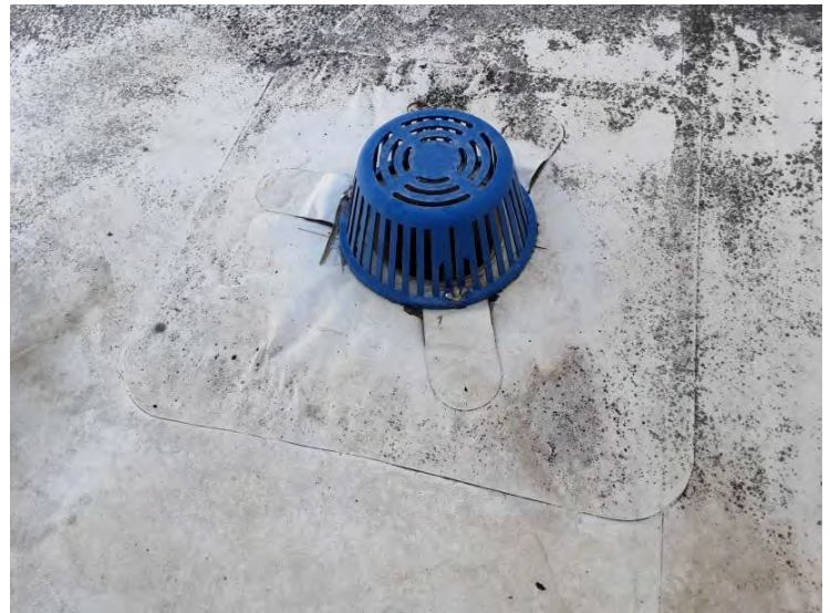
South TPO Roof - Roof Drains Roof drains appear to be in fair condition.
