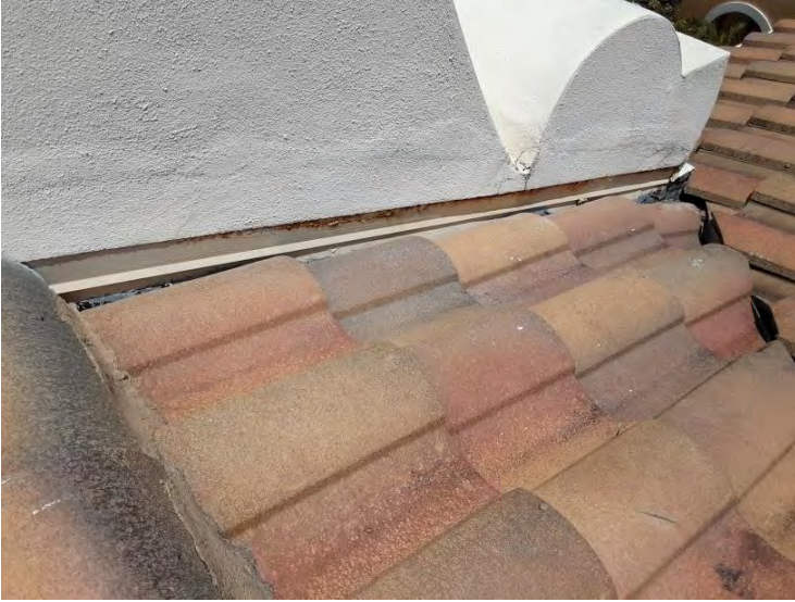
Center Tile Roof - Counter Flashings
