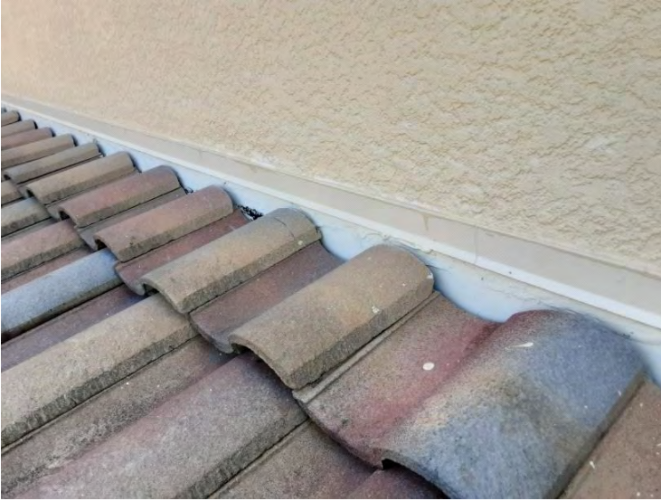
South Tile Roof - Counter Flashings
