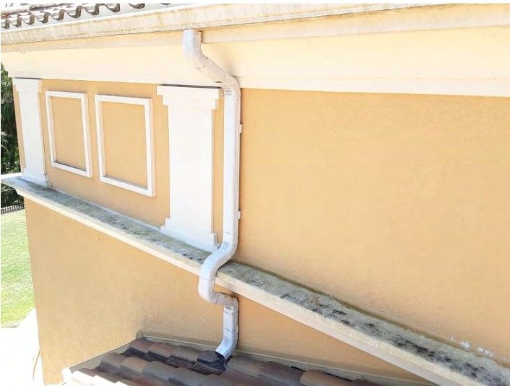
Center Tile Roof - Downspouts The downspouts appear to be in fair condition.
