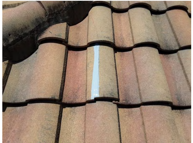
North Tile Roof - Field Tiles - Completed Repair
