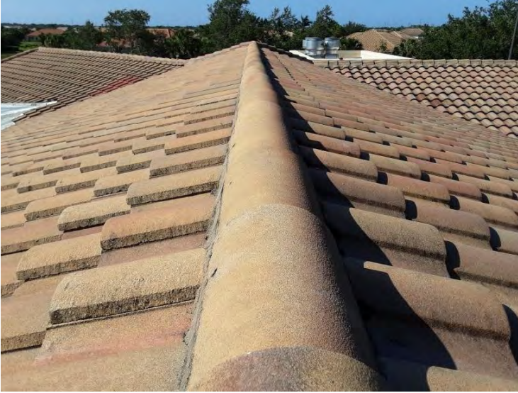
South Tile Roof - Ridge Tiles Ridge tiles appear to be in fair condition.
