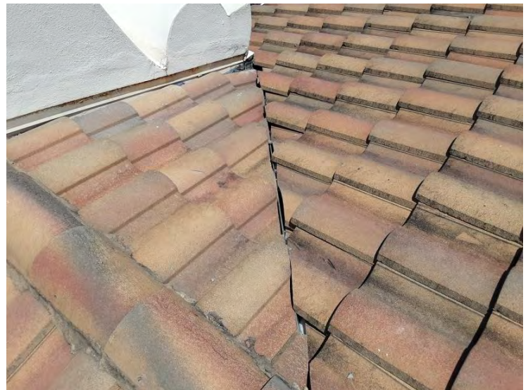
Center Tile Roof - Ridge Tiles Ridge tiles appear to be in fair condition.
