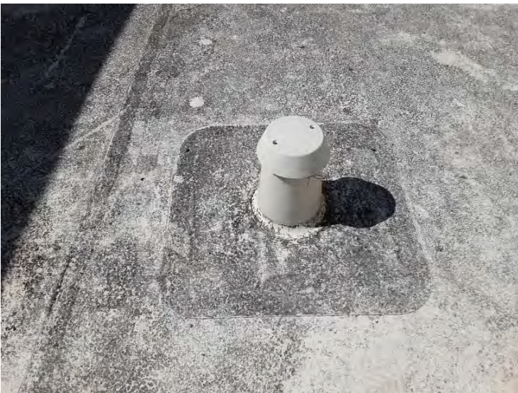
South TPO Roof - One Way Vent One way vent appears to be in fair condition.
