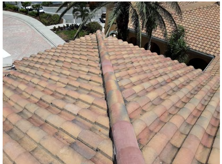
Center Tile Roof - Hip Tiles Hip tiles appear to be in fair condition.
