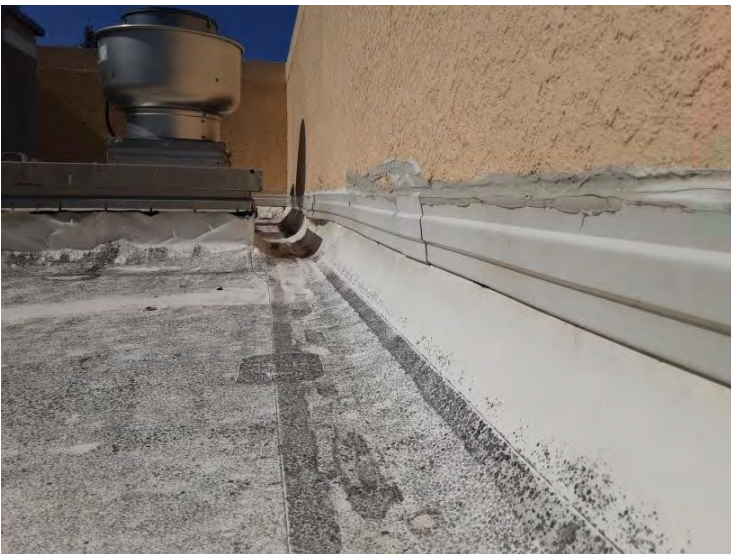
South TPO Roof - Base Flashings
