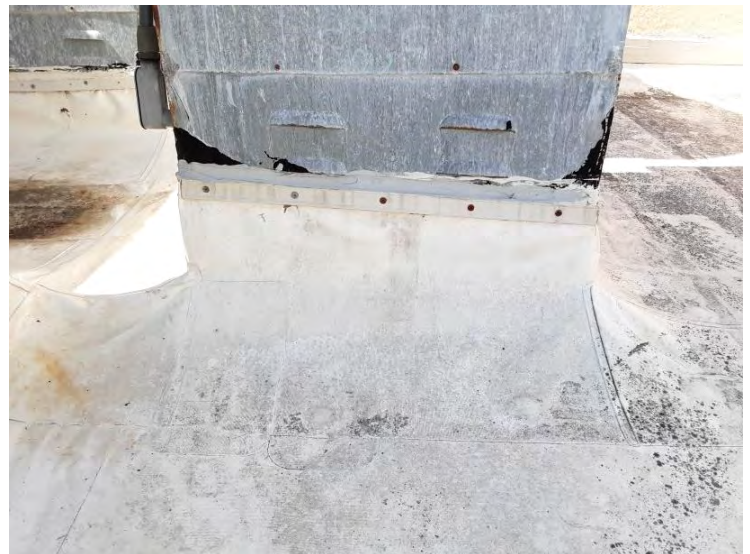
South TPO Roof - Roof Vent Base Flashings Roof vent base flashings appear to be in fair condition.
