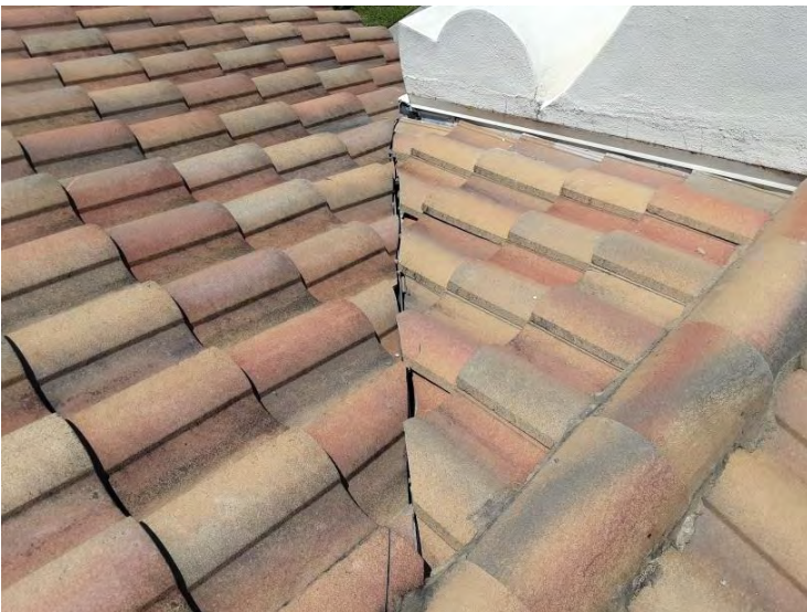
Center Tile Roof - Valley Tiles Valley tiles appear to be in fair condition.
