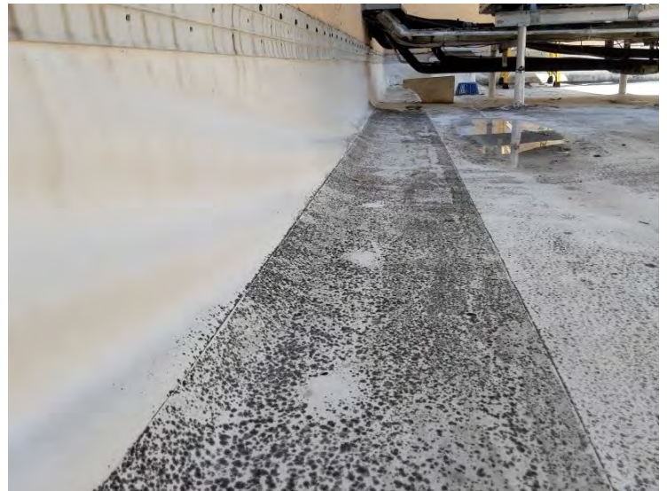
North TPO Roof - Base Flashings
