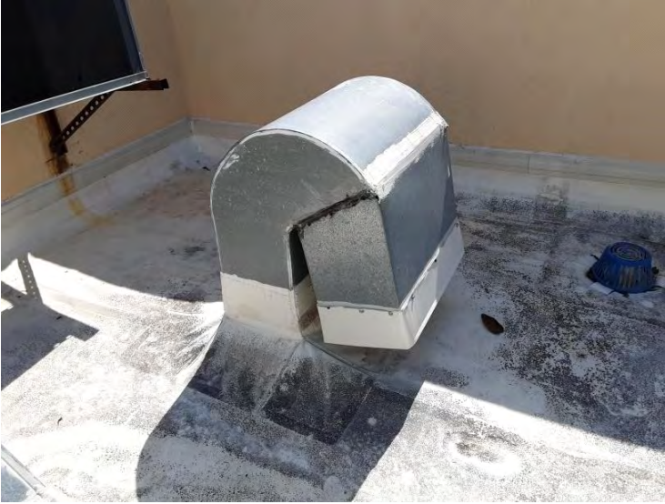
South TPO Roof - Roof Vents Roof vent appears to be in fair condition.
