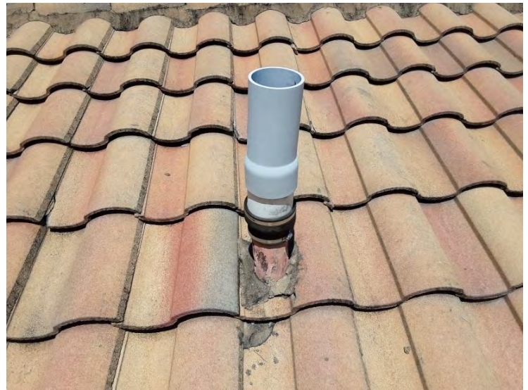
North Tile Roof - Lead Boots Lead boots appears to be in fair condition.
