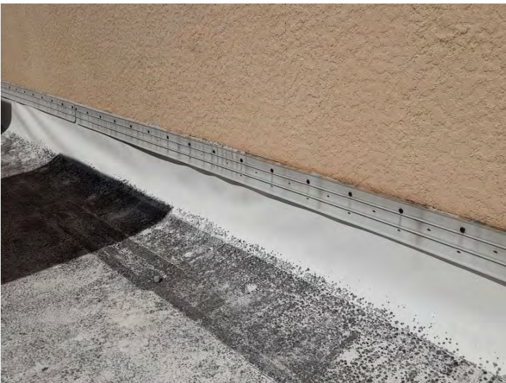
North TPO Roof - Counter Flashings
