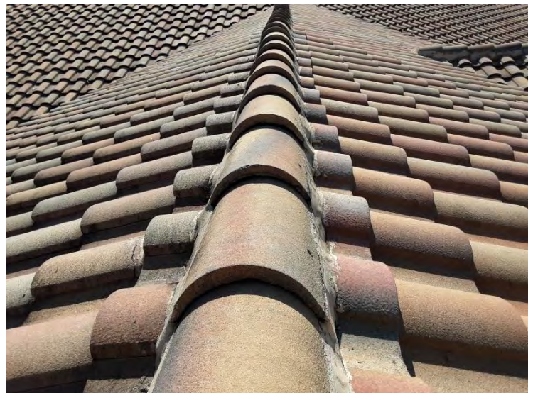
South Tile Roof - Ridge Tiles Ridge tiles appear to be in fair condition.
