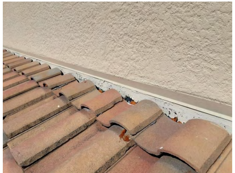
South Tile Roof - Counter Flashings
