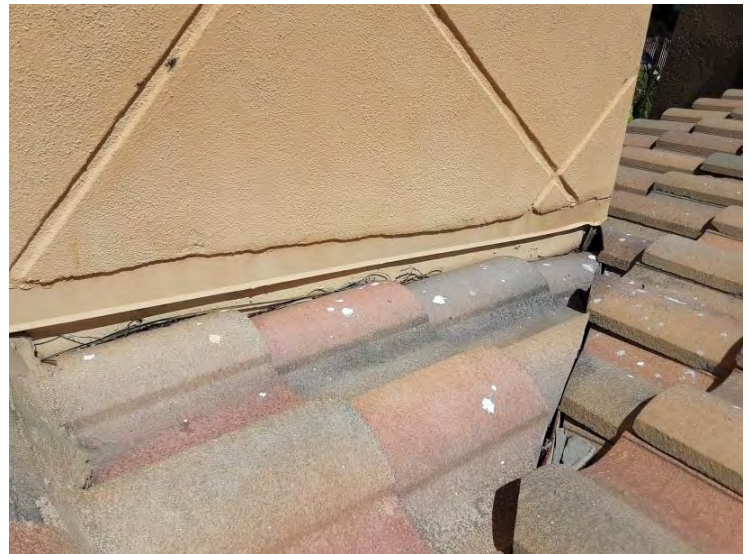
North Tile Roof - Counter Flashings
