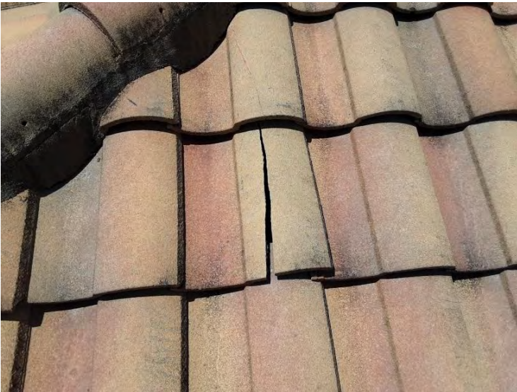
North Tile Roof - Field Tiles - Damaged Tiles
