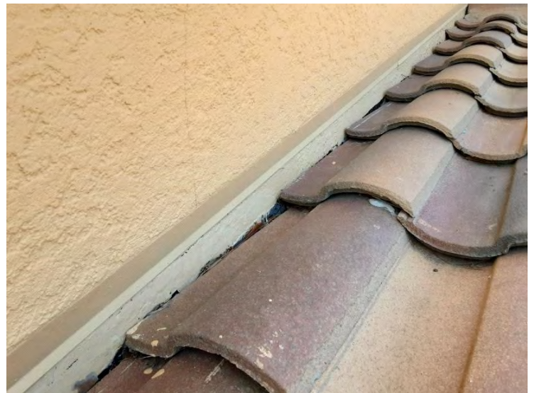
North Tile Roof - Counter Flashings
