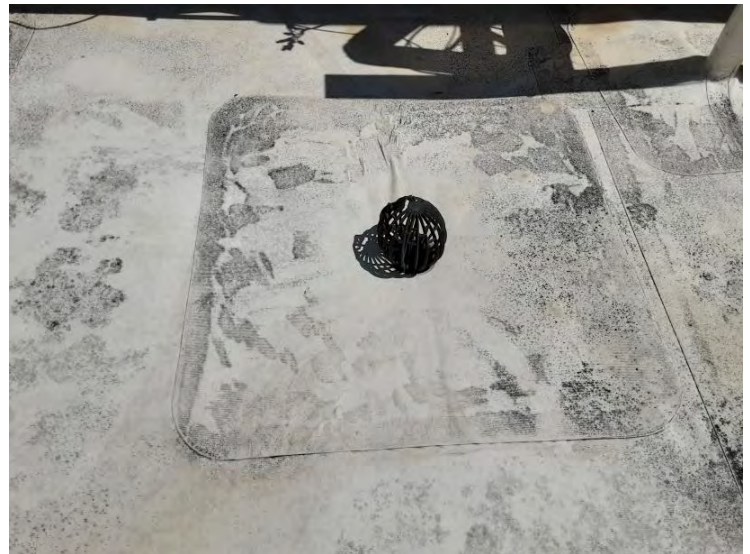
North TPO Roof - Roof Drains Roof drains appear to be in fair condition.
