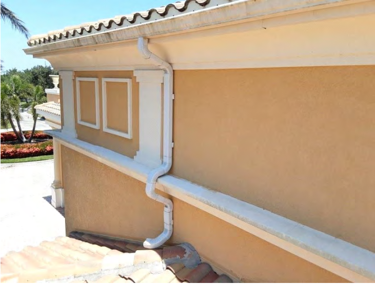
Center Tile Roof - Downspouts
