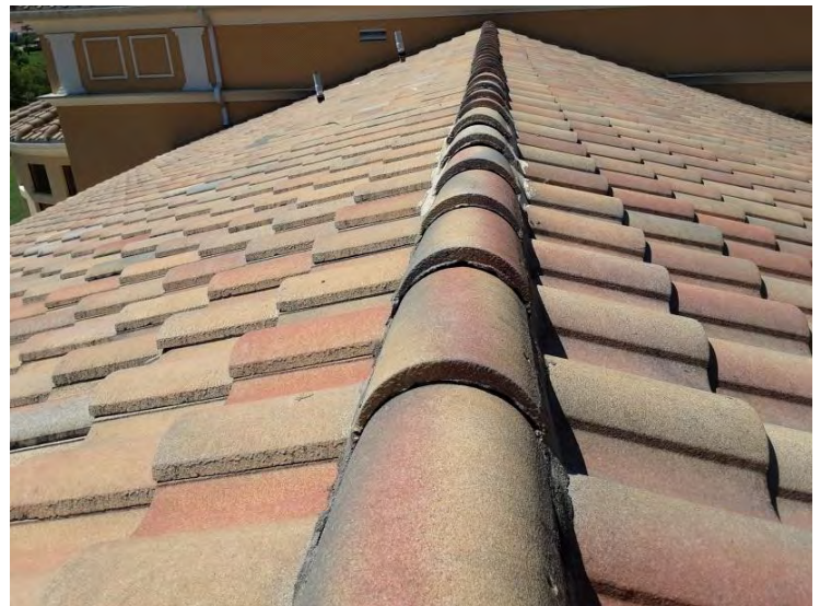
North Tile Roof - Ridge Tiles
