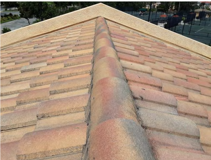
North Tile Roof - Ridge Tiles
