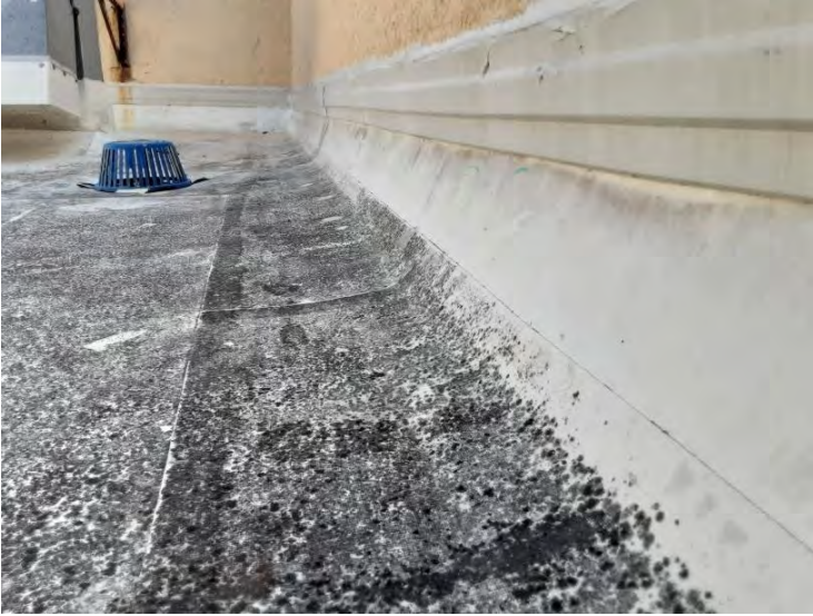
South TPO Roof - Base Flashings
