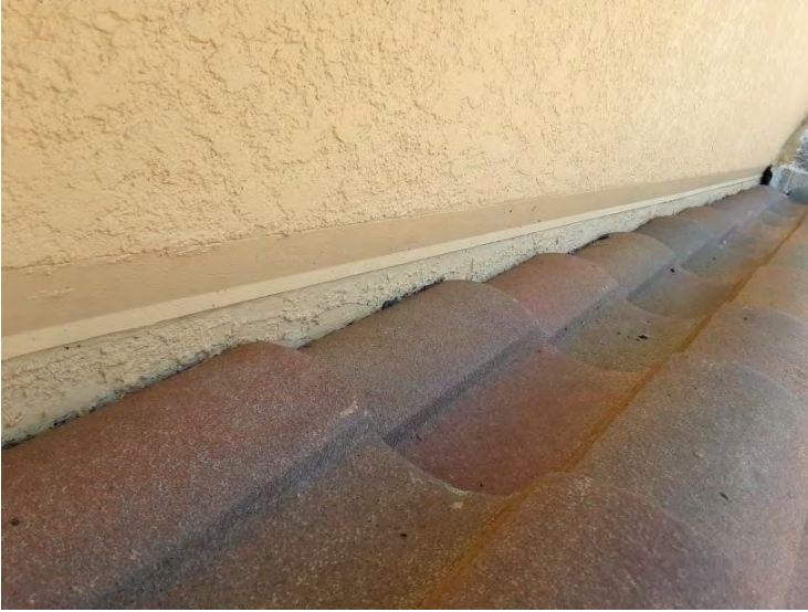
North Tile Roof - Counter Flashings
