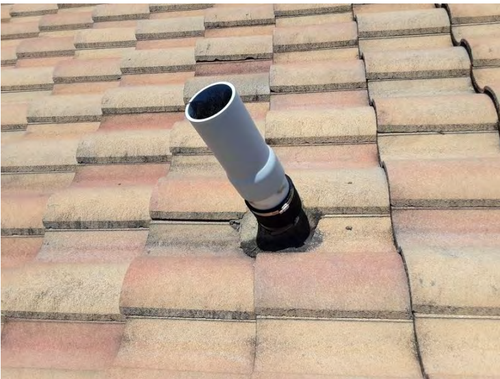
North Tile Roof - Lead Boots ??? PVC Boot Lead boots appear to be in fair condition.
