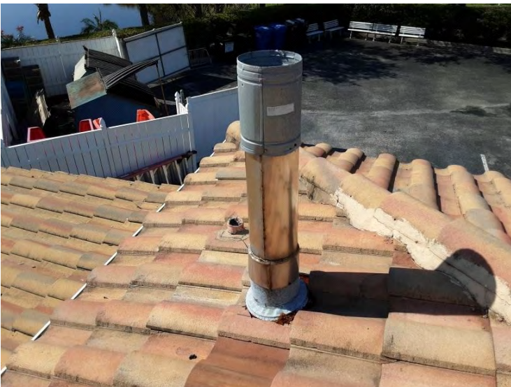
South Tile Roof - Roof Vents Roof vent appear to be in fair condition. Crowther Roofing identified roof vent loose strap and missing cover.
