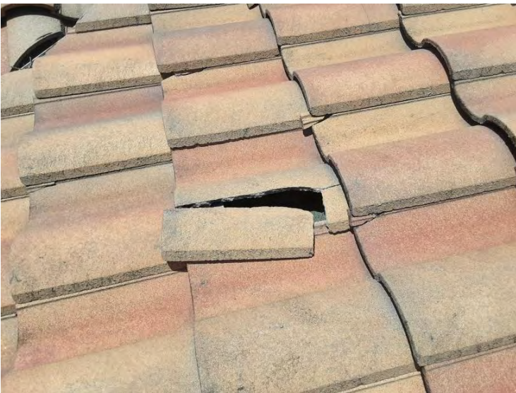
North Tile Roof - Field Tiles - Damaged Tiles
