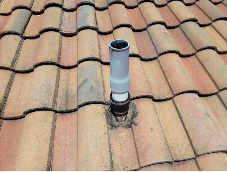
North Tile Roof - Lead Boots Lead boots appear to be in fair condition.
