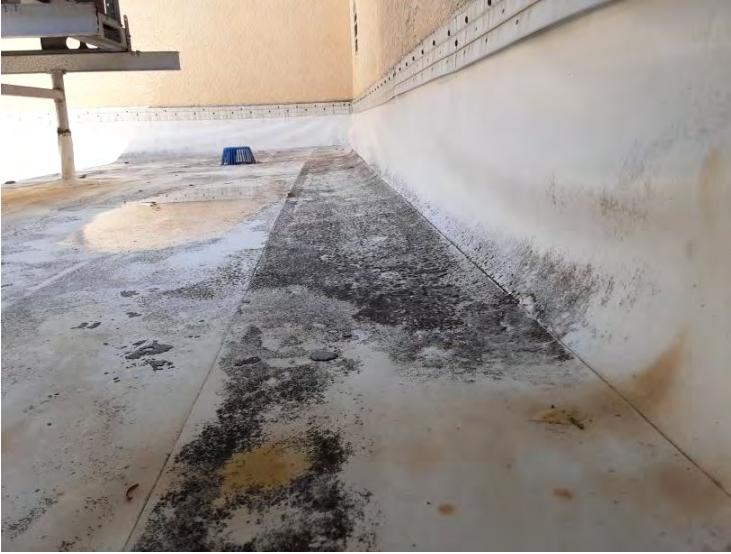
North TPO Roof - Base Flashings
