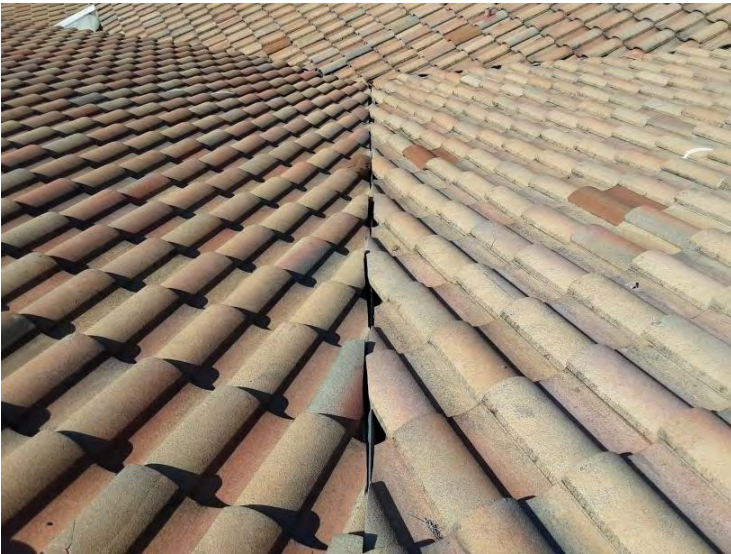
South Tile Roof - Valley Tiles Valley tiles appear to be in fair condition.
