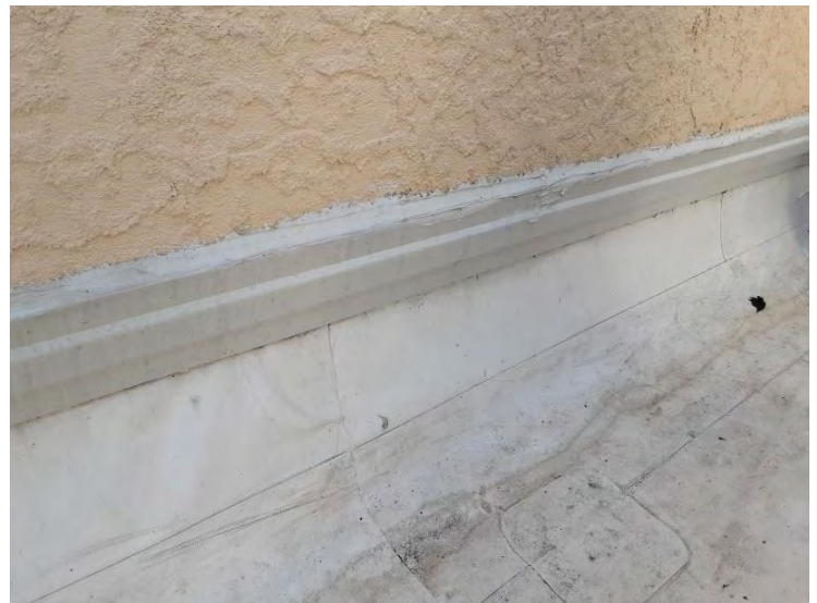
South TPO Roof - Counter Flashings
