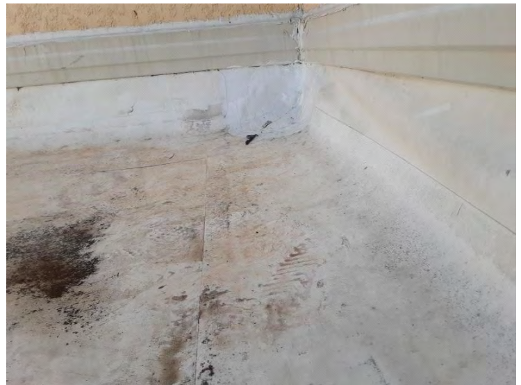
South TPO Roof - Base Flashings
