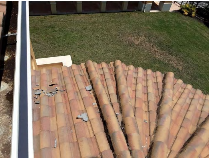
Center Tile Roof - Field Tiles - Damaged Tiles
