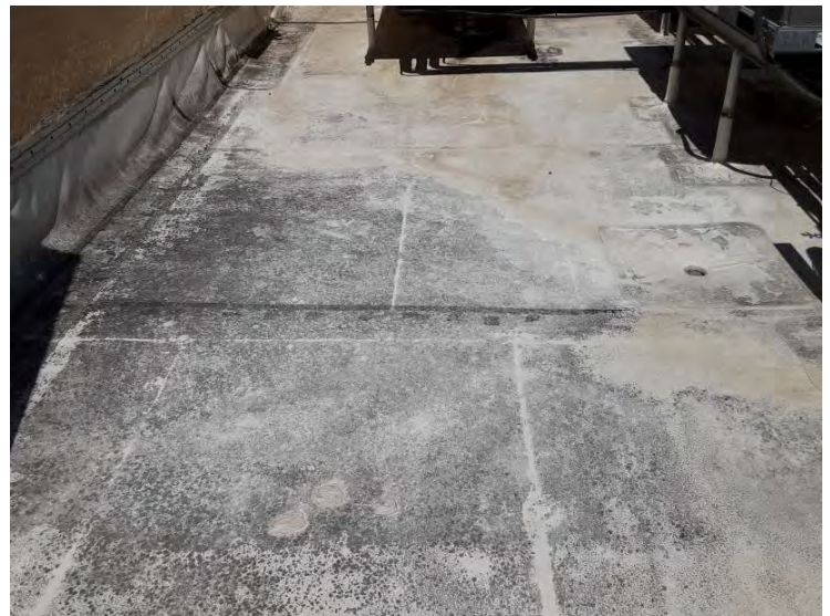
North TPO Roof - Membrane Overview The roof membrane appears to be in fair condition.
