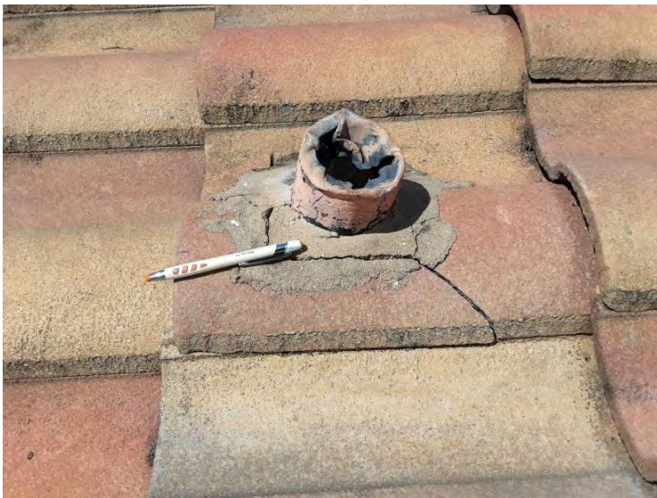
South Tile Roof - Field Tiles - Damaged Roof Tile Identified damaged roof tile that can allow premature underlayment deterioration from excessive UV exposure.
