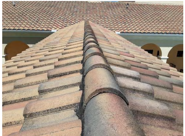
North Tile Roof - Ridge Tiles Ridge tiles appear to be in fair condition.
