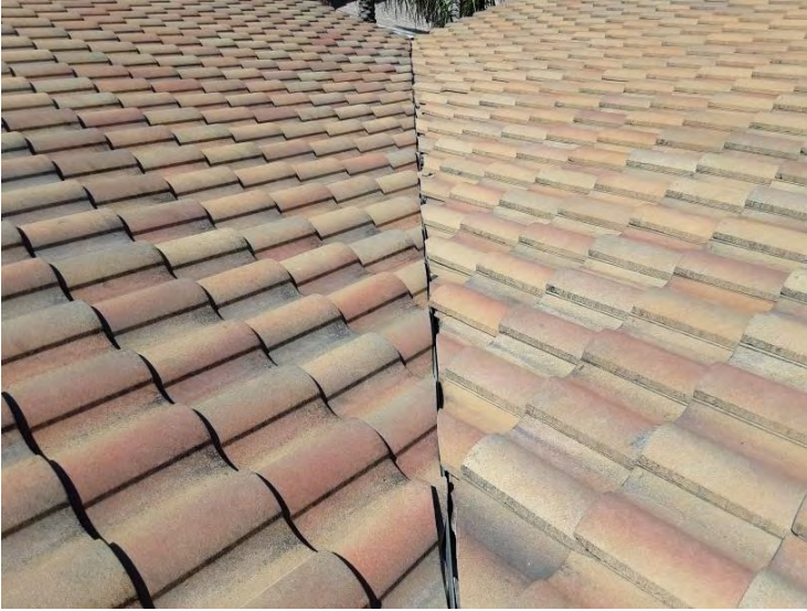
North Tile Roof - Valley Tiles Valley tiles appear to be in fair condition.
