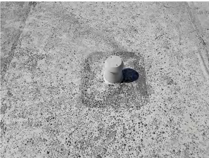
Center TPO Roof - One Way Vent
